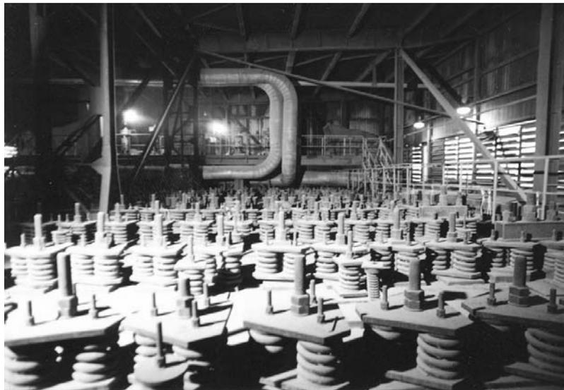
Figure-1. Elastic suspensions of boiler.
